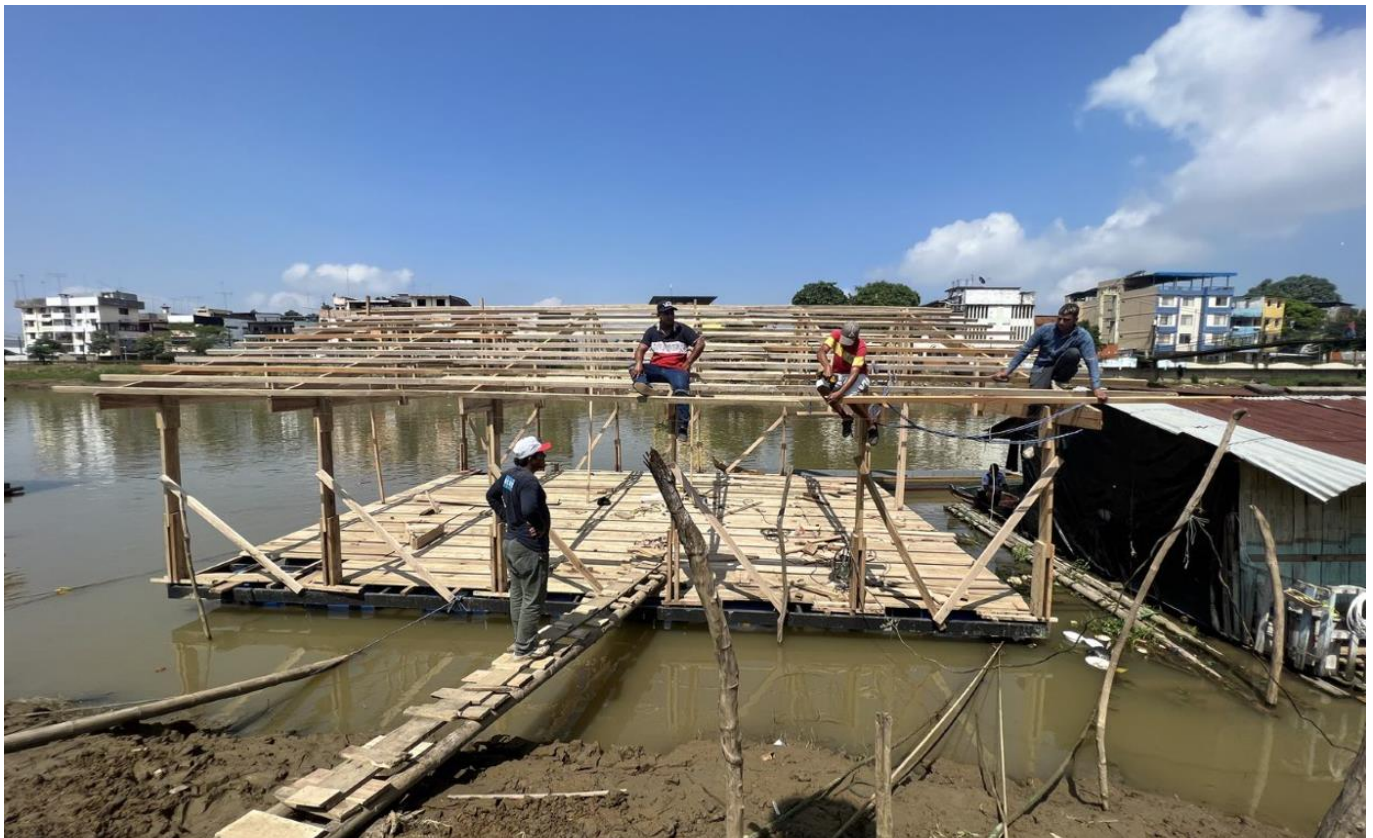
Placement of wooden structural roof - "La Balsanera - Floating Productive House". Credit: © Natura Futura.
